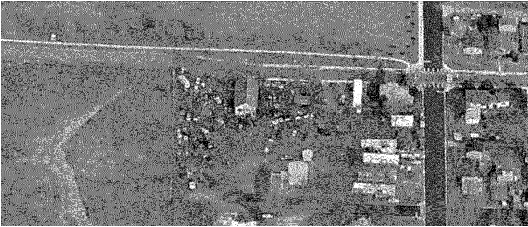
Figure 3: Condition of subject lots prior to the Marshall Fire
