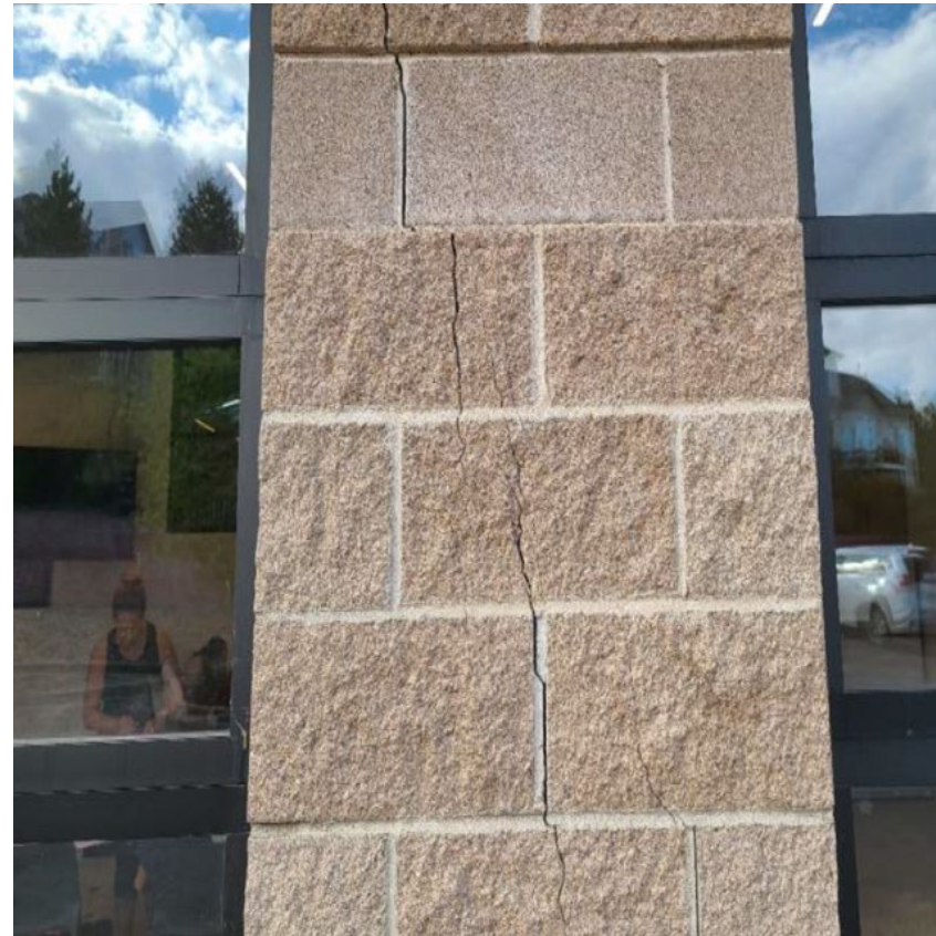
Masonry Cracking
