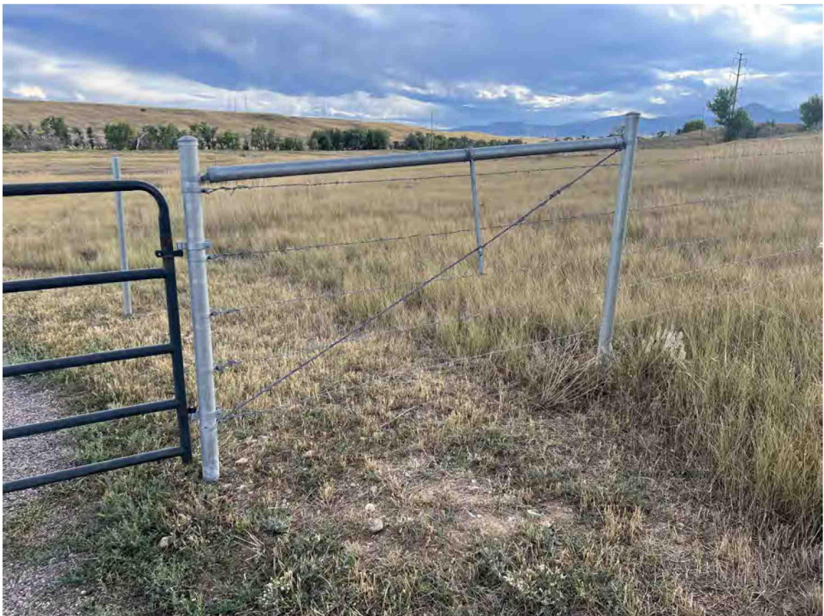
E C4.0 STEEL TENSIONING POSTS - REFERENCE IMAGE
