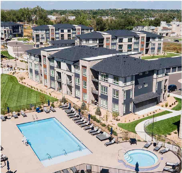
POOL & SPA DECK
