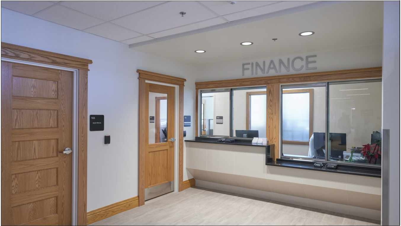
Enclosed Finance service counter, protected by a Level 3 bullet-resistant window and wall system. Each public counter has a duress button.
